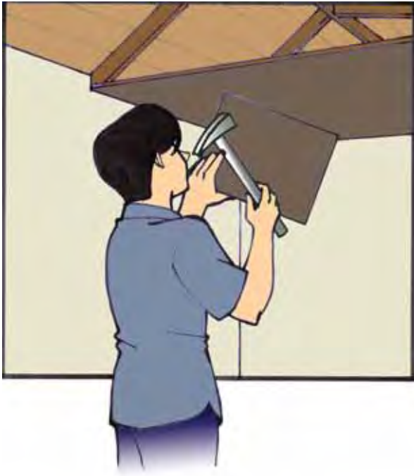
Figure 61: Installing a ceiling is an effective way to reduce heat penetration from outside.
